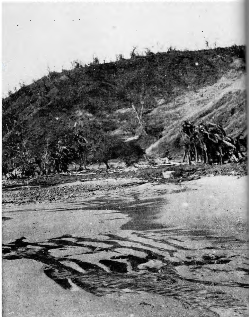
All that was left of the stone breakwater and receiving shed — nothing
